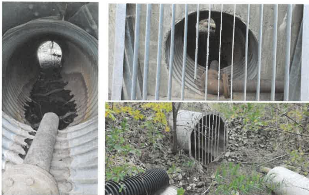
Photograph #2 – Current Central Pond Outlet
